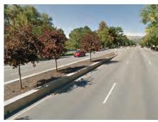
Raised center median with left turn bays for turning traffic on 700 East near Liberty Park in Salt Lake City Construct a hard- or greenscaped raised median to replace the existing paint-striped center turn lane. Leave gaps for left turning motorists to enter major destinations and adequate entrances for left turning motorists
