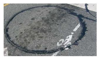
Standard loop detection pavement marking (Photo: NACTO)
